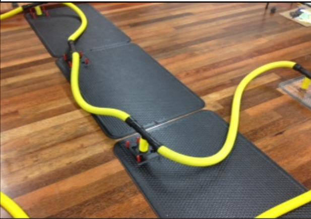
Before placing the Vac-It Panels onto the surface to be dried, remove all standing water. Place Panels onto the surface but do not place tape on the Panels at this time.
