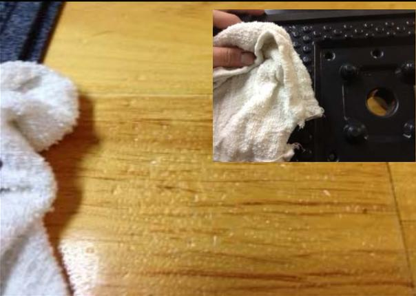
Now extract the floor for at least 30 minutes. Lift the panels occasionally to wipe away any visible liquid that may have pooled under the panels (on bottom of panel and on top of flooring). Extract until there is no more bulk liquid coming from flooring.
