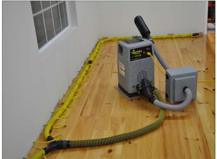
Injectidry's High Pressure drying systems are specifically developed to target high risk areas of hidden moisture such as: walls and ceilings, even those coated with watertight finishes like PVA paint and vinyl wallpaper coverings, double-sheeted fire walls, party walls, sound barriers, insulation, walls behind cabinets and fixtures and floors.
