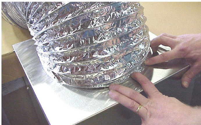
Figure 5: Inlet ducting
